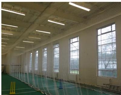
*The lights had been aligned with the playing lanes. This did not provide good illumination to walls so 'cave-effect' was visible due to the poorly-lit walls.*
