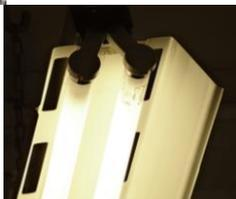
*We saw that the existing T8 tubes were halophosphate and this, combined with starters and magnetic ballasts, led to a situation where light-levels dropped significantly through the life of the tubes. They were also quite yellowed, and the colour-rendering was only Ra60, and these factors combined to make the hall feel dingy.*
