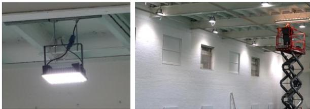
We felt that the best choice would be our lights with Philips LEDs which provide luminaire efficiency of 130lm/watt. We did not want to go to very cool daylight as we felt this would be too shocking a transformation but milder 5500k did refresh the hall compared to the former T8 halophosphate tubes. We also agreed the walls needed painting to improve reflectance.
